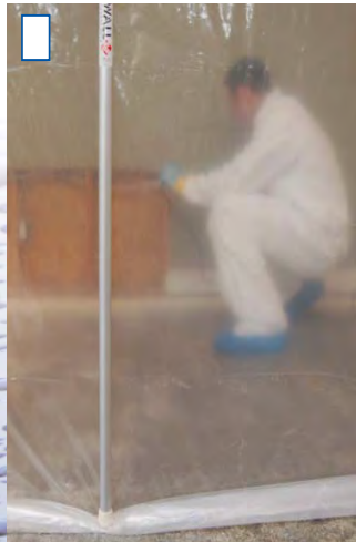
STEP 5: Set up Lead Containment, if applicable.
