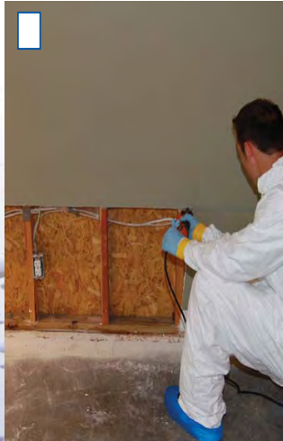
STEP 6: Remove affected baseboards and dry wall.
