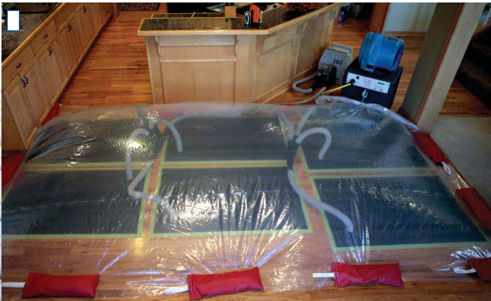
STEP 5: Tent & duct in dehumidified or dry-heated air.
