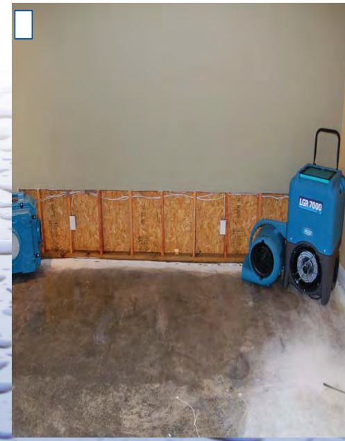
STEP 10: Install equipment.
