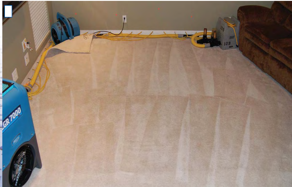
STEP 3: Dry carpet, pad and structure. (Floating)
