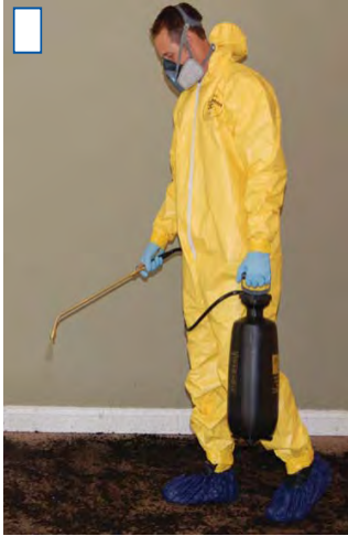
STEP 1: Apply initial disinfectant.
