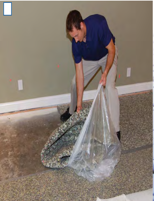
STEP 3: Remove damaged pad.
