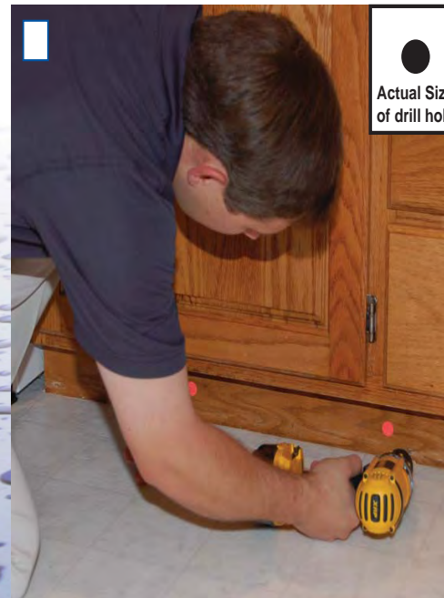
STEP 3: Drill drying ports.
