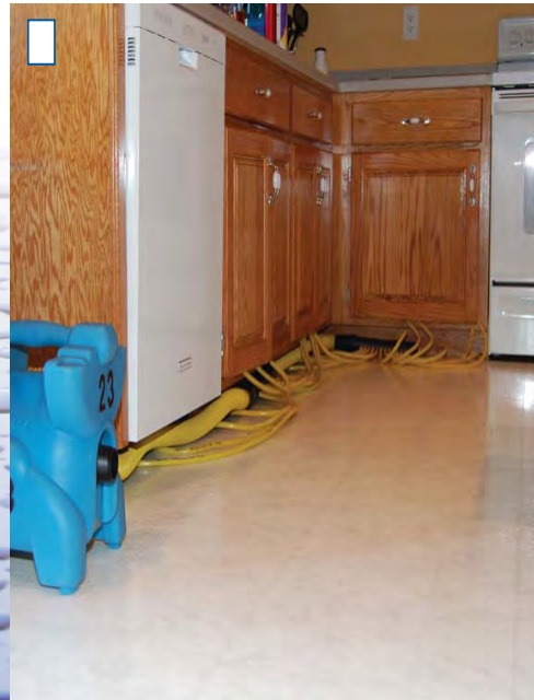
STEP 8: Dry cabinets and walls.
