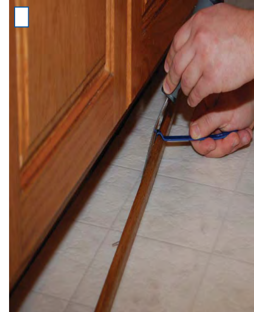
STEP 4: Install injectors into toe kick.
