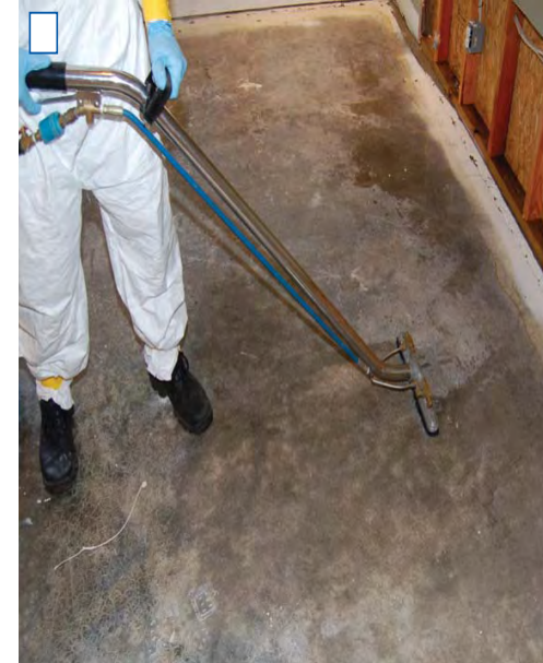
STEP 8: Steam clean.
