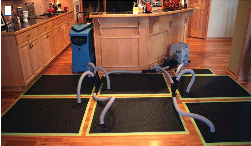
STEP 4: Secure hoses and install drying equipment.
